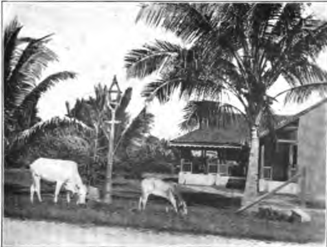
REST HOUSE AT KWALA KANGSAR
